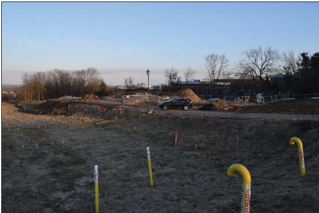
Photograph 4: Study Area as observed from the northwest corner of the site.
