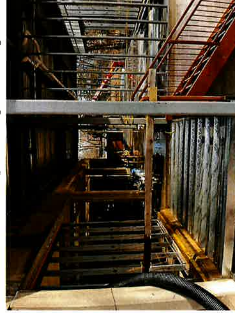
Interior Framing and Rough-In in Progress
