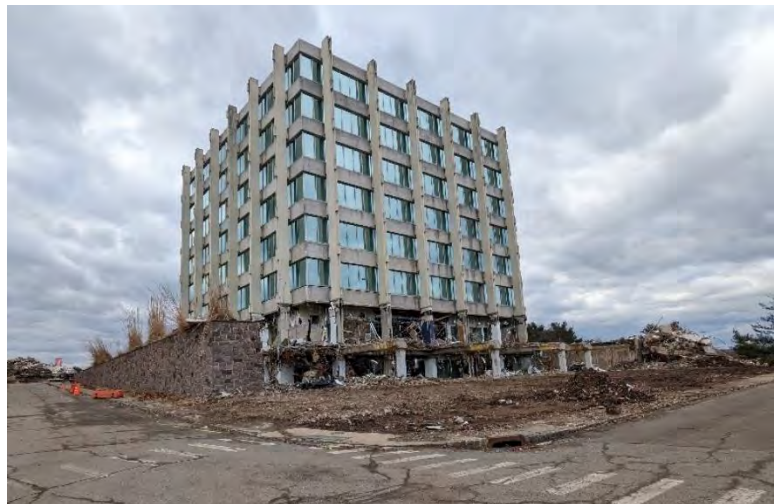
FIGURE 2: NORTHWEST STRUCTURE BEING DEMOLISHED FOR THE PROPOSED WAREHOUSE FACILITIES (1/26/23).
